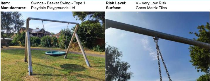
Finding: Swings of this design should have a secondary Action: Monitor use and check the joint and fixing security safety mechanism fitted to prevent collapse of the seat in the regularly event of a joint failure to comply with BS EN 1176 Part 2, however this swing was installed prior to the standards being updated in 2018 and the manufacturer has confirmed that the joint was independently cycle tested by BSi
