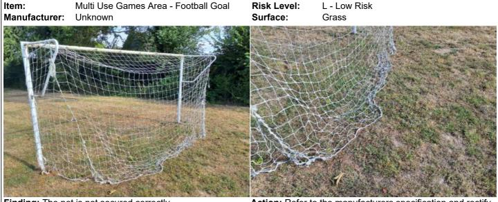
Finding: The net is not secured correctly
